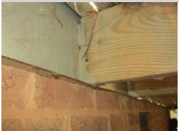
The metal hangers used to support the floor framing of the deck were installed without the proper number and sized nails. The nail installation is crucial to the function of the hanger, without proper installation the hanger could fail allowing the deck to move or collapse. A licensed general contractor should be consulted for complete evaluation of the deck and to make necessary repairs.
