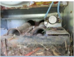
The gas burner section of the package unit has visible rust and debris in the burner chamber area. The rust indicates deterioration of the exchanger. Deterioration of the heat exchanger is a serious concern that can result in improper combustion and carbon monoxide poisoning. The furnace needs a complete evaluation which should include a heat exchanger inspection to ensure safe, reliable, and proper operation of the HVAC system. A licensed HVAC contractor should be consulted for repair.
