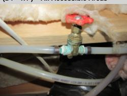
The main water supply line located in the crawl space at the back door is corroded. Corrosion on the main water lines should be addressed as soon as possible to prevent major leaks and property damage. A licensed plumbing contractor should be consulted for a complete evaluation and repair of the main water supply line.
