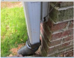
Additional Photograph: This a photograph of a decayed vertical trim molding behind the back left gutter.
