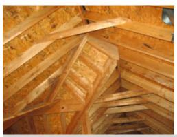
From the attic, it was noted that the Valley/Hip rafter located between the main home and first floor room was not posted for end support. End post supports are typically installed to supplement nailed joints and ensure the stability of the roof system. An engineer should be consulted for further evaluation to determine the significance and cause of the concern and outline necessary repairs to ensure the stability of the structure.
