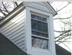
The trim cladding along the roof rake / eave was not formed to provide a lip to support the shingles and prevent water from traveling behind the trim. A siding installation company or general contractor should be consulted to evaluate and repair the trim to ensure the integrity of the cladding system.
