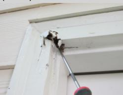
The door has extensive soft and decayed wood in the frame area . Decay in the door frames can result in leaking and water penetration and should be repaired as soon as possible. A general repair specialist or licensed general contractor should be consulted for evaluation and repair.
