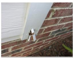
The exterior trim of the home need repairs and painting to prevent further damage and water penetration. The following items were noted during the inspection all areas should be evaluated as a repair plan is prepared:
