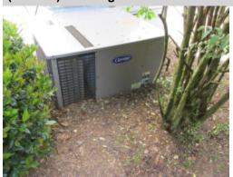
The grading around the package HVAC unit is directing drainage toward the unit. Evidence suggests that water from lot drainage has been entering the unit., see next photograph. Drainage needs to be corrected to prevent damage to the unit. A licensed general contractor should be consulted for further evaluation and repair.
