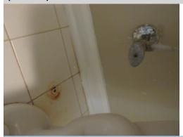
The floor area under the toilet tank has a rust stain indicating a history of a leak or a seeping leak at the tank bolts or water turn off. The toilet tank bolts/gaskets and the turn off valve need to be evaluated by a plumber to ensure that they are not leaking. A licensed plumbing contractor should be consulted for evaluation and repair.
