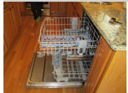
The dishwasher is not secure to the cabinet and it moves forward when the door is opened. The appliance needs to be secured to the cabinet to prevent damage to the unit or personal injury. An appliance repair person or general contractor should be consulted for repair.
