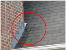
The gutter downspout at the right dormer is not extended or piped out to direct roof drainage away from the side wall of the main home. Direct drainage from the gutter system can result in direct water penetration into the attic areas of the home. A licensed general contractor should be consulted for a complete evaluation and to make necessary repairs.
