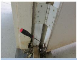
Additional Photograph: The door also has soft and decayed wood in the door panel area. Decay in the door panel can result in leaking and water penetration and should be repaired as soon as possible. A general repair specialist or licensed general contractor should be consulted for evaluation and repair.
