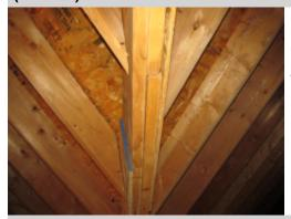
From the attic, it was noted that the valley rafter located over the main living room was constructed of multiple members and was not posted for support. Post supports are typically installed to supplement nailed joints and ensure the stability of the roof system. An engineer should be consulted for further evaluation to determine the significance and cause of the concern and outline necessary repairs to ensure the stability of the structure.
