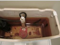
The toilet flush valve is not operating properly. This could result in improper functioning, flooding and waste of water. A licensed plumbing contractor should be consulted for evaluation and repair.
