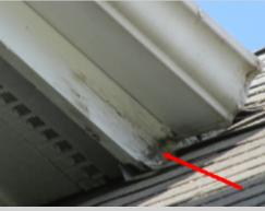
The exterior boxing of the home need repairs and painting to prevent further damage and water penetration. The following items were noted during the inspection all areas should be evaluated as a repair plan is prepared:
