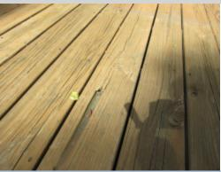
The wood deck was found to be severely weathered. Decking boards were splintering and cupped. The deck should be considered hazardous. A licensed general contractor should be consulted for complete evaluation of the deck and to make necessary repairs.
