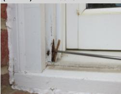
The all windows have soft and decayed wood in the sill, trim, sash areas. Decay in the windows can result in leaking and water penetration and should be repaired as soon as possible. All windows should be inspected for similar damage as repairs are made. A licensed general contractor should be consulted to evaluate the extent of the damage and make necessary repairs.
