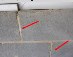
Closed cracks were noted in the foundation of the garage at locations where the foundation steps related to elevation change. Cracks in the foundation indicate a deficiency in the foundation, footing, or supporting soil that can change and worsen if it progresses over the life of the home. An engineer should be consulted to determine the significance /cause of the cracks and outline any necessary repairs.
